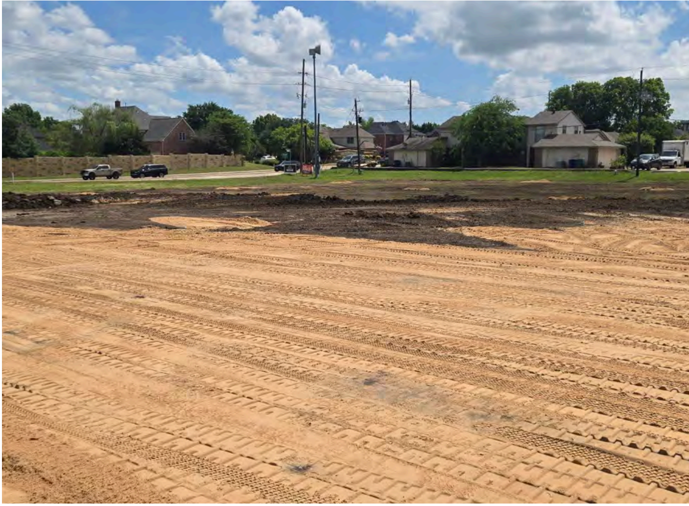
CHANDLERS LANDING FIELD RENOVATION
