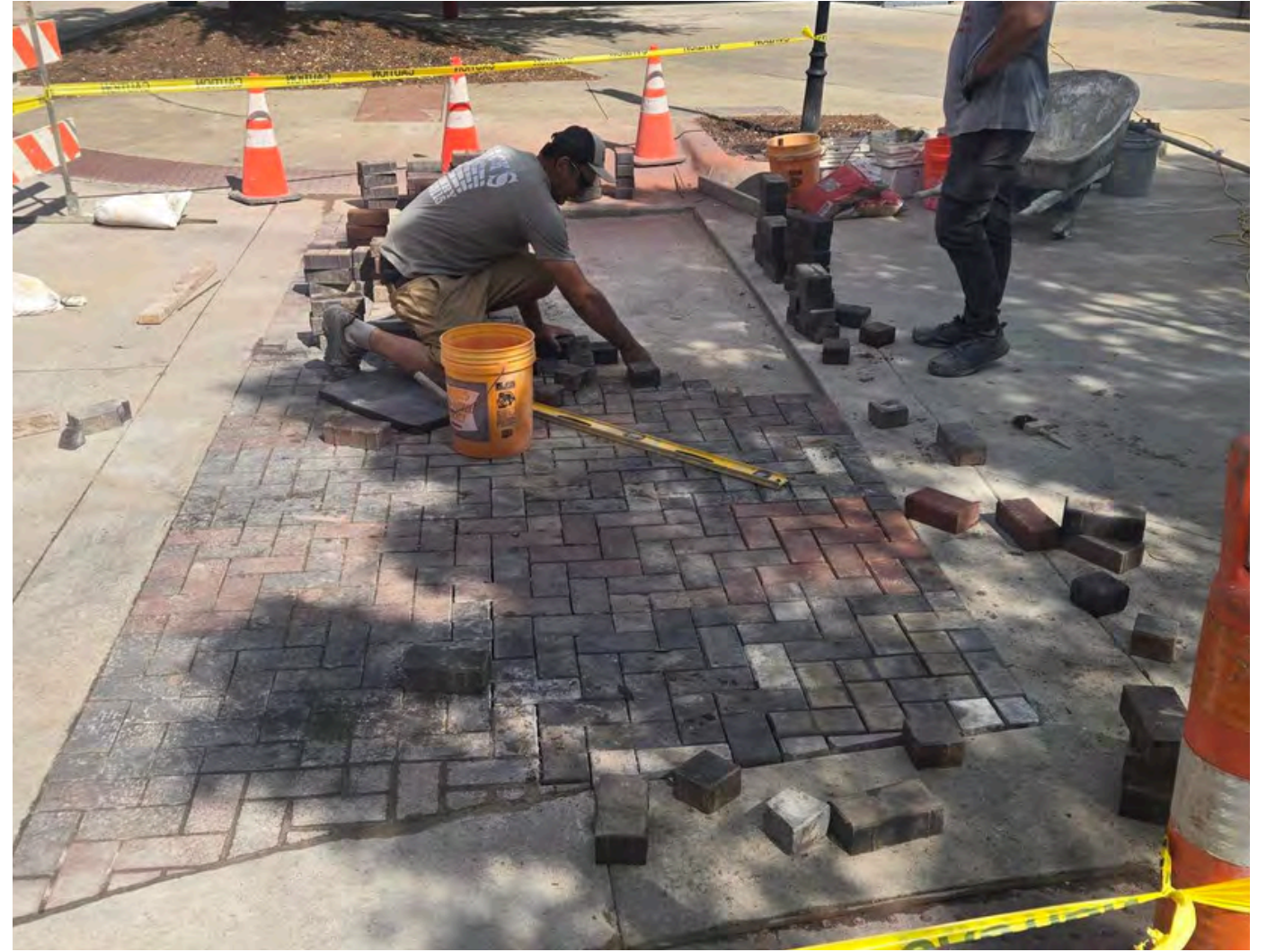
DOWNTOWN CROSSWALK REPAIRS
